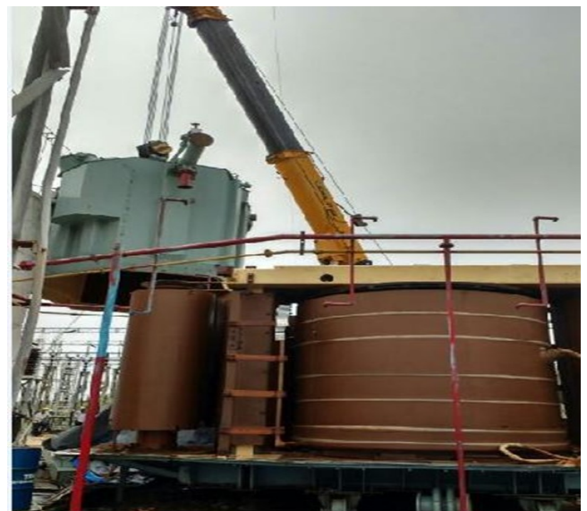
Fig. 11. Inspection of active part of transformer
