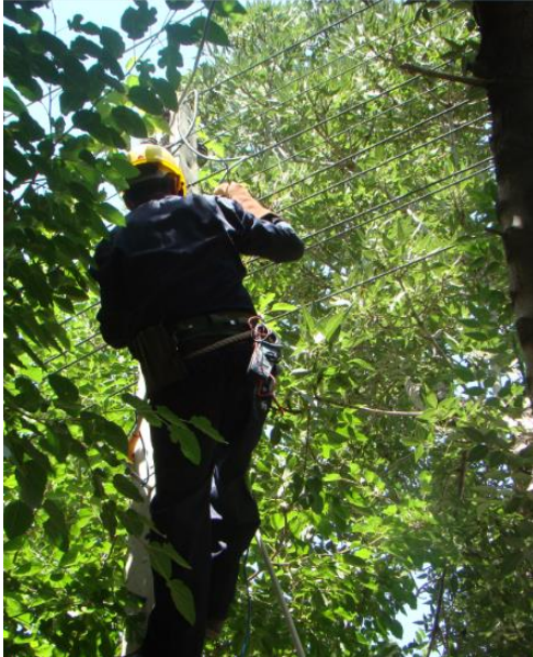
Fig. 2. Limb's direct connection to S-phase of 380 volt network (Ash tree)
