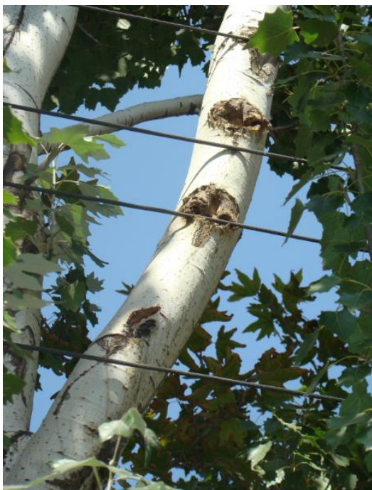
Fig. 1. Constant contact of Plane tree with low voltage network, Hamedan/Iran.
